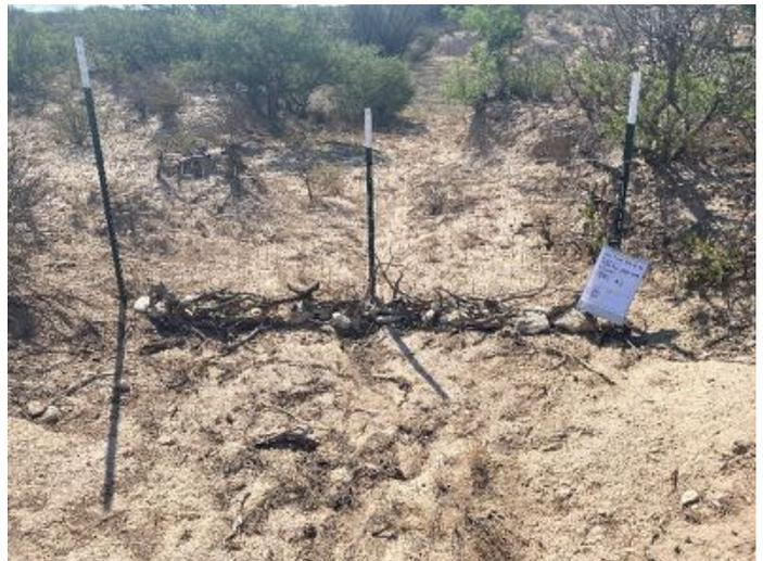
**Figure 9.** One of twenty erosion control structures installed along headcuts of the Black River.
