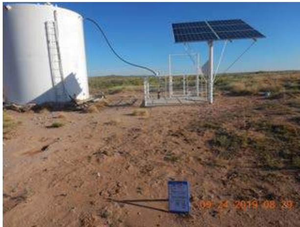
**Figure 3.** Solar Pump Installed Next to an Existing Storage Tank.
