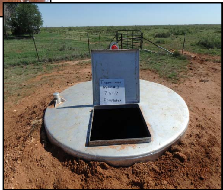
Figures 1 & 2: Completed Pithouse & Submersible Pump
