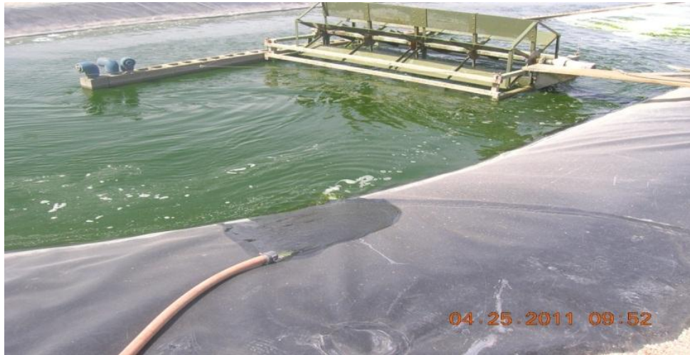
Figure 5. Supernatant returned to source pond.
