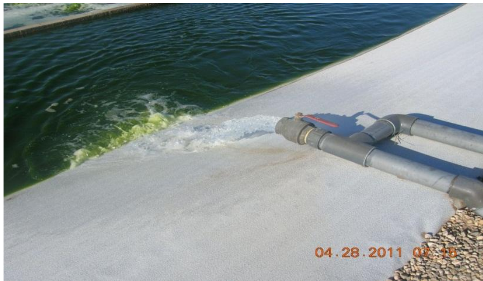
Figure 6. Fresh water from a ground water source added to attain proper salinity.
